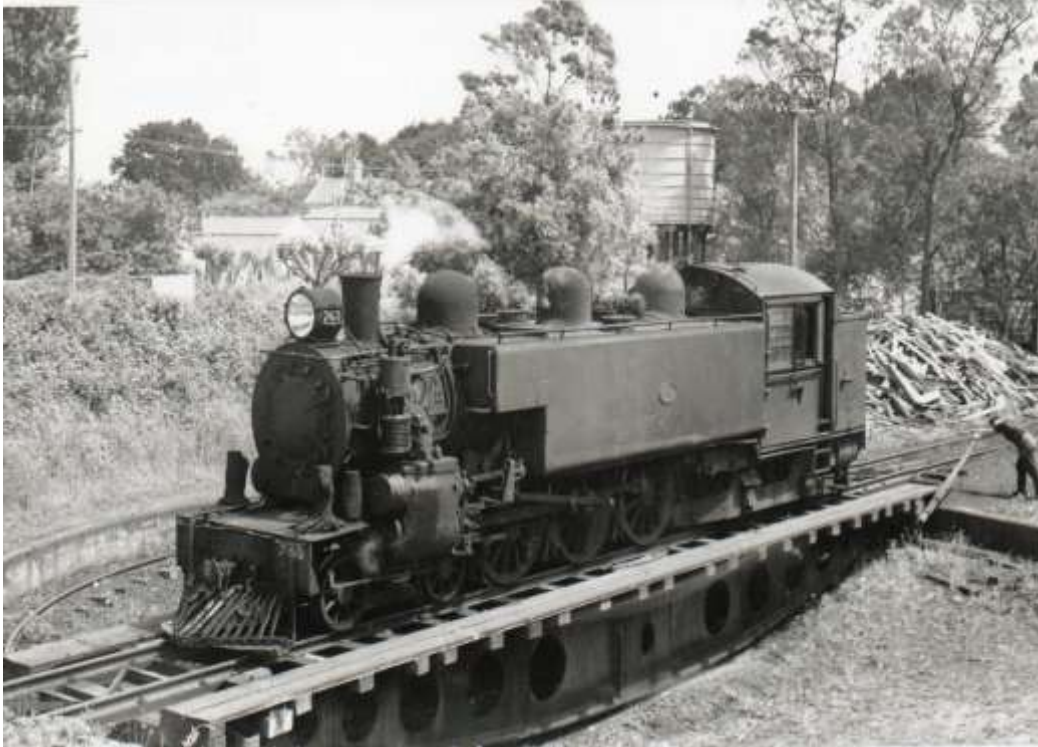
Turntable and water tank, railway house in rear. Papakura Museum 19159P
